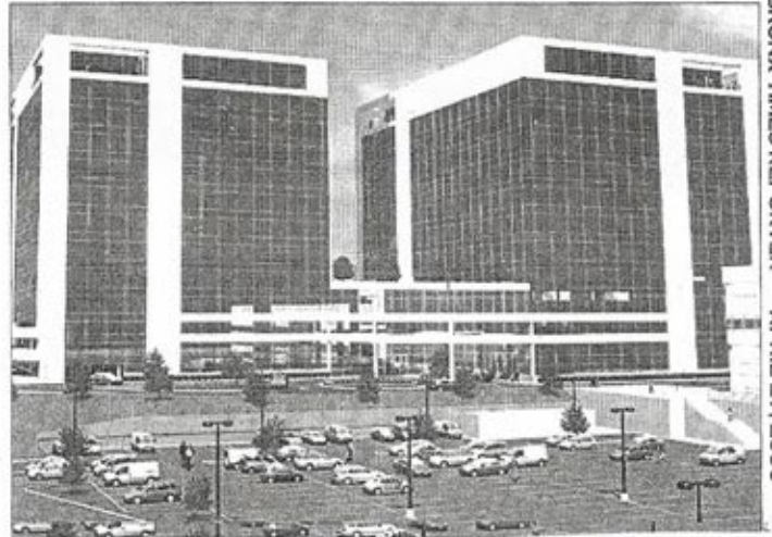
(Right) Good news abounds at the Hutchinson Metro Center. The Towers (pictured) are planned for this year at the Waters Place office complex, while its Class A office space is nearly fully leased.
